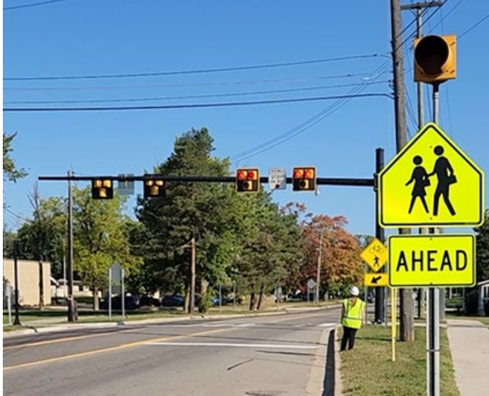
Figure 5: HAWK Signal Along Wixom Road
