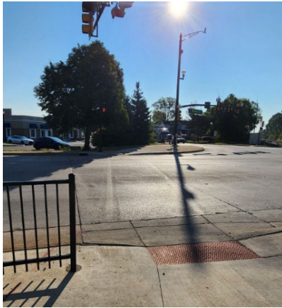
Figure 16: Faded crosswalk at the Wixom Road and Pontiac Trail intersection
